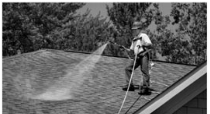
Apply Roof Maxx Protection
