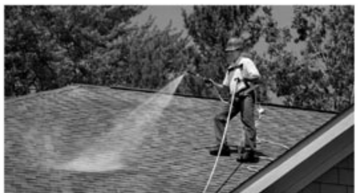
Apply Roof Maxx Protection
