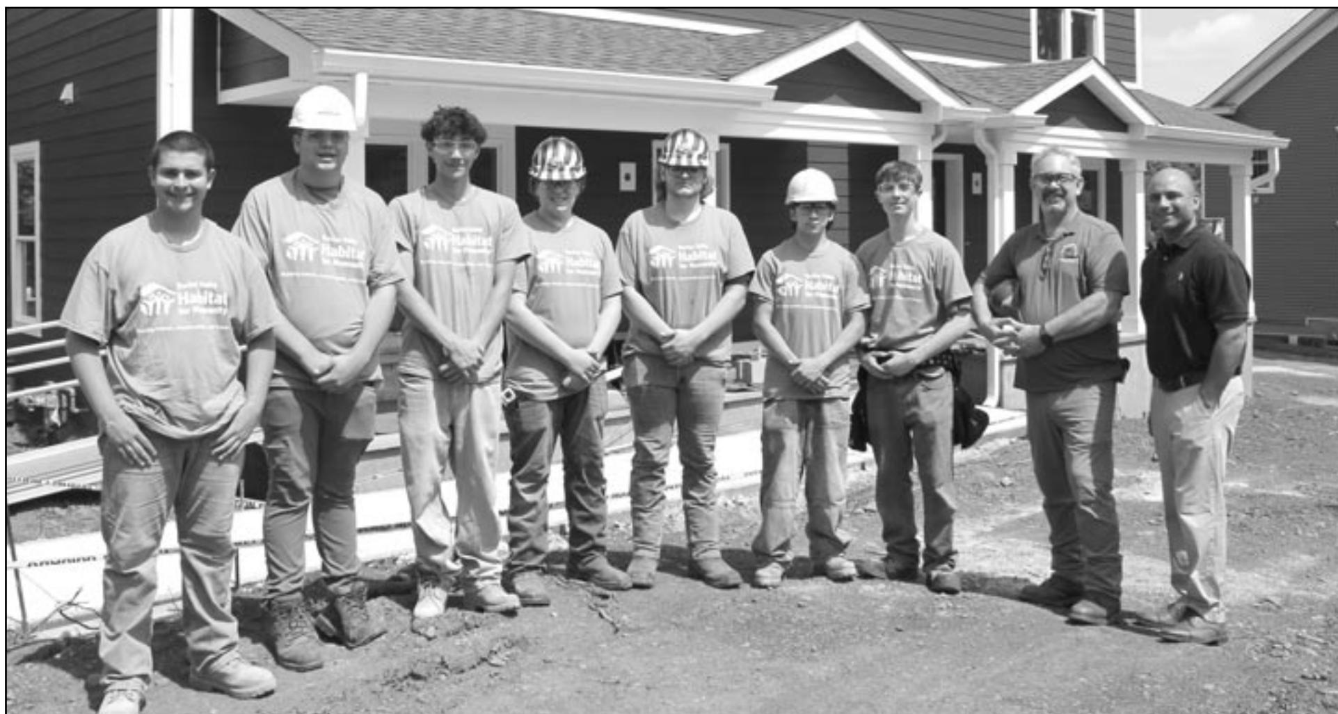
(above, l-r) SCVTHS staff and students joined Raritan Valley Habitat for Humanity at a worksite in Whitehouse Station. Pictured are Ryan Phelan of Hillsborough, Antonio DiMonte of Bridgewater, Ben Canuso of Manville, Logan Rice of Branchburg, Nick DeSan of Bound Brook, Kyle Tobar of Manville, George Bittman of Bridgewater, SCVTHS Carpentry Instructor Dan LaRue, and SCVTHS Supervisor of CTE Robert Carrig.
