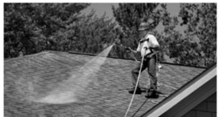
Apply Roof Maxx Protection
