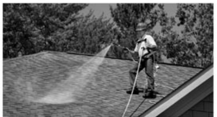
Apply Roof Maxx Protection
