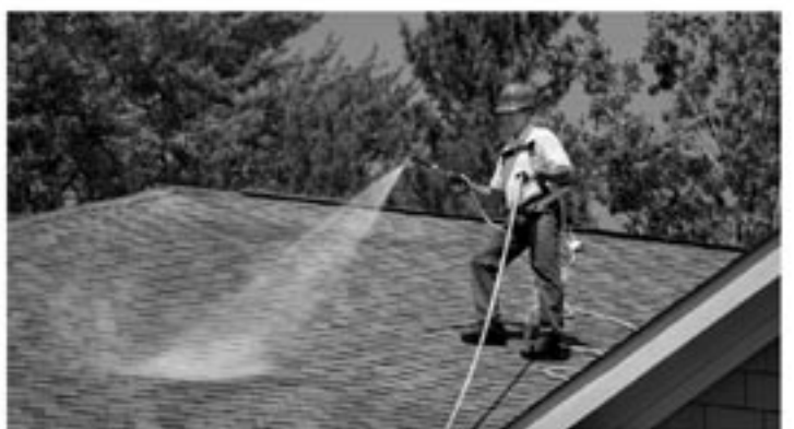
Apply Roof Maxx Protection
