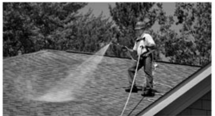
Apply Roof Maxx Protection
