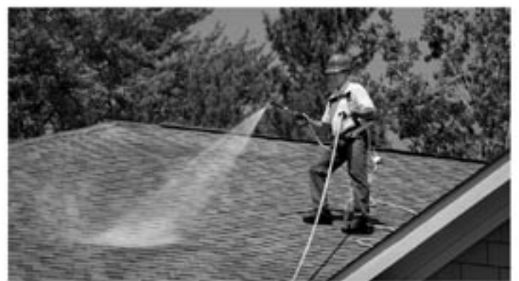
Apply Roof Maxx Protection
