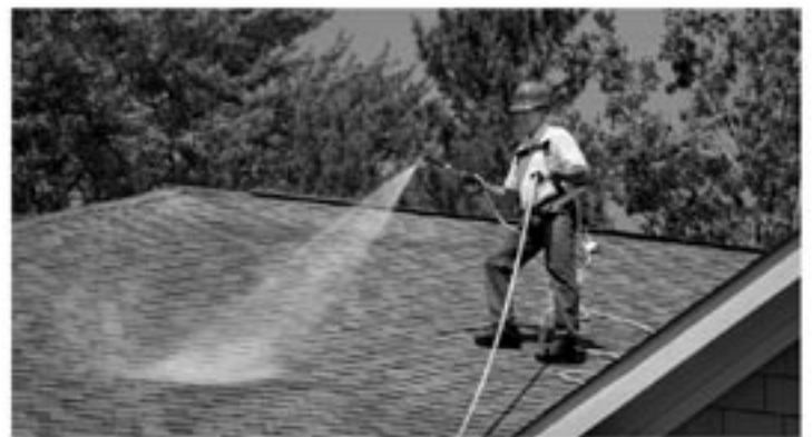
Apply Roof Maxx Protection
