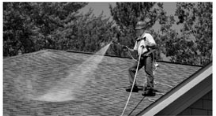
Apply Roof Maxx Protection
