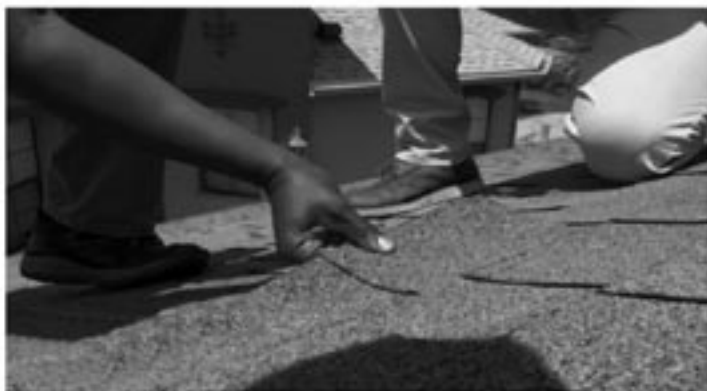
FREE Inspection and Estimate
