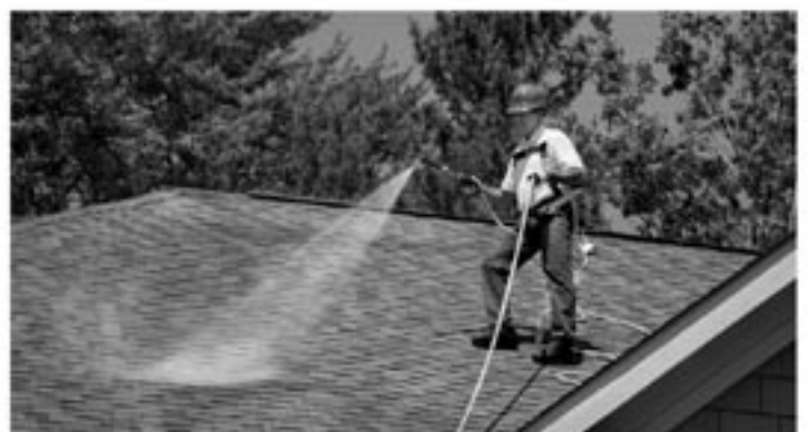
Apply Roof Maxx Protection
