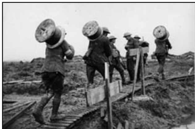
Laying communications lines in France made easier due to the presence of duckboards. The muddiness of the terrain required the mass construction of miles of these simple narrow wooden walkways both above ground, and also in the elaborate mazes of trenches that dominated the countryside.
