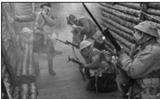
A typical scene inside a WWI trench outfitted with advanced construction. Wood lines the walls and floors, keeping the soldiers more comfortable and above the wet ground that made trench foot a common, debilitating condition of the infantry soldier. Note that each soldier is equipped with a gas mask, a standard part of a WWI issued gear.
