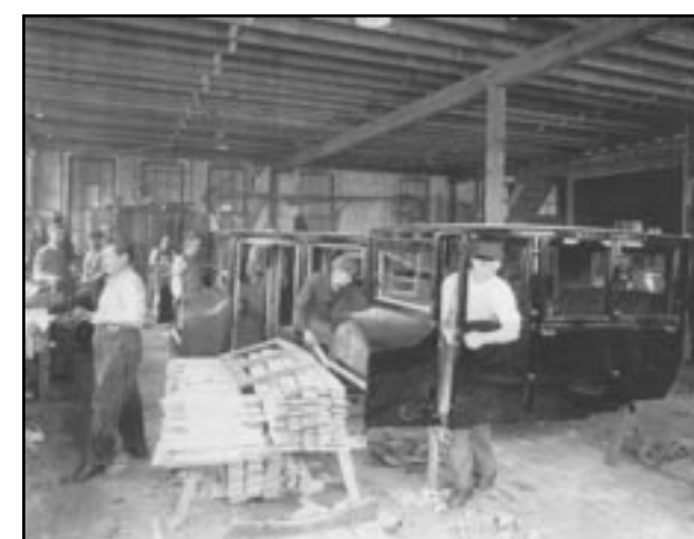
(above) Automobile bodies taking shape as doors, glass, and hardware are fitted.
