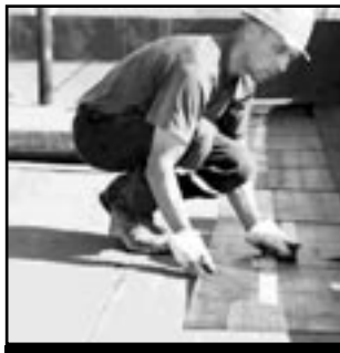
FLAT TOP ROOF
