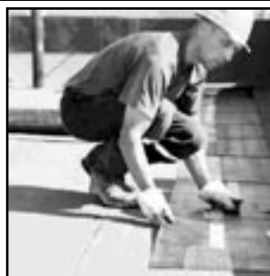
FLAT TOP ROOF
