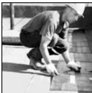
FLAT TOP ROOF
