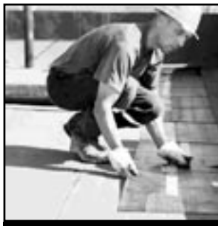
FLAT TOP ROOF
