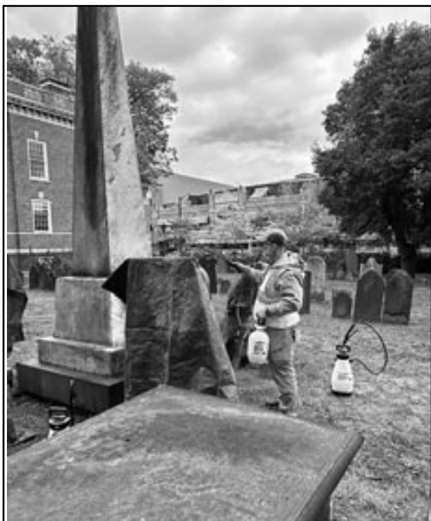
(above) The recent restoration and cleaning of the James and Hannah Caldwell Memorial Obelisk at Siloam-Hope First Presbyterian Church in Elizabeth was commissioned by the Union County Historical Society.
