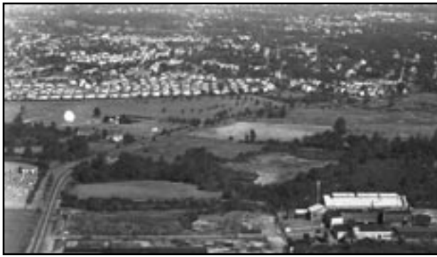
(above) Industrial building bottom right corner is site of today's Kenilworth Inn Hotel. Two square areas at center are farm land, part of Merck site today.
