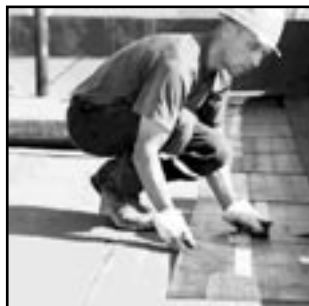
FLAT TOP ROOF
