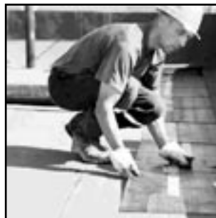
FLAT TOP ROOF
