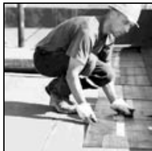
FLAT TOP ROOF
