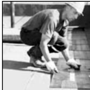
FLAT TOP ROOF
