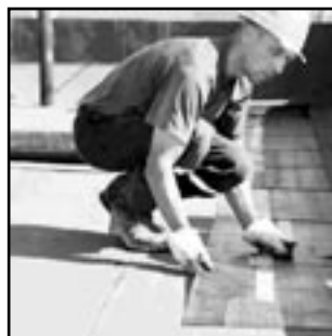
FLAT TOP ROOF
