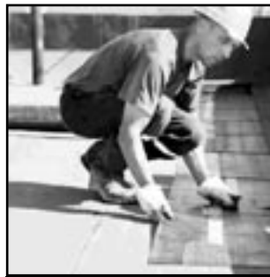
FLAT TOP ROOF
