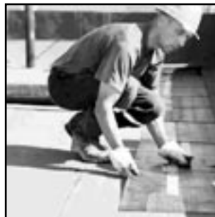
FLAT TOP ROOF
