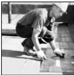
FLAT TOP ROOF
