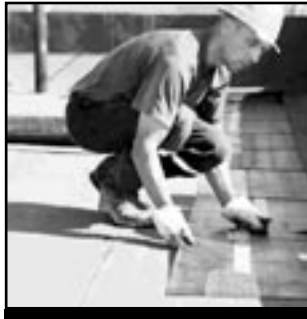
FLAT TOP ROOF
