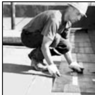
FLAT TOP ROOF
