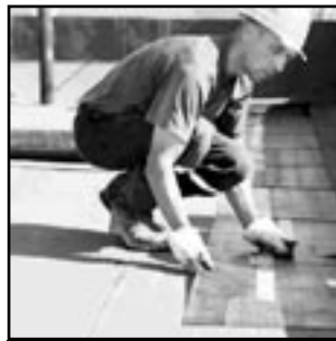
FLAT TOP ROOF
