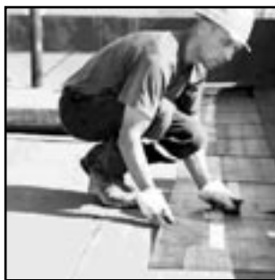
FLAT TOP ROOF
