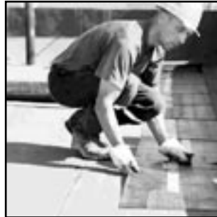
FLAT TOP ROOF
