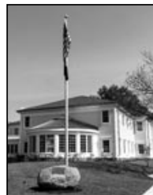
(above) Library exterior
