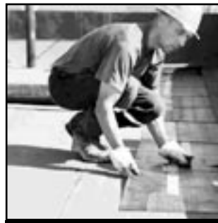
FLAT TOP ROOF
