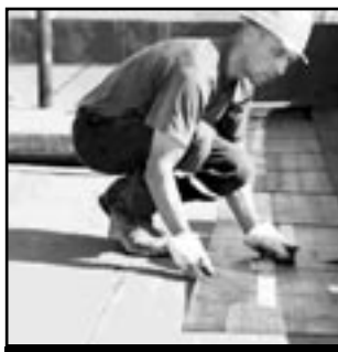
FLAT TOP ROOF
