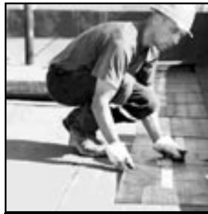
FLAT TOP ROOF
