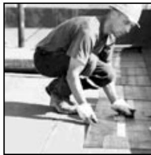
FLAT TOP ROOF
