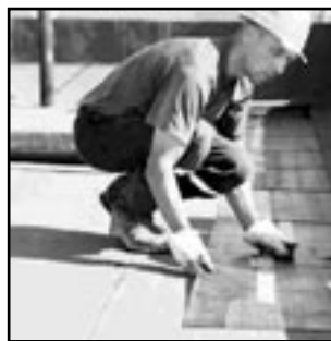
FLAT TOP ROOF
