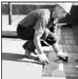
FLAT TOP ROOF
