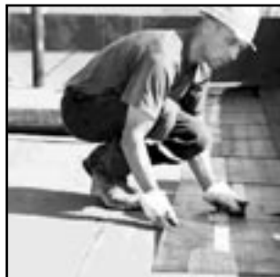
FLAT TOP ROOF
