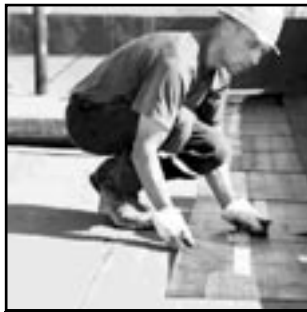
FLAT TOP ROOF
