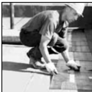
FLAT TOP ROOF
