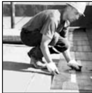
FLAT TOP ROOF
