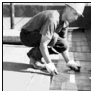
FLAT TOP ROOF
