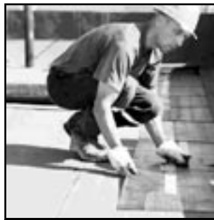
FLAT TOP ROOF
