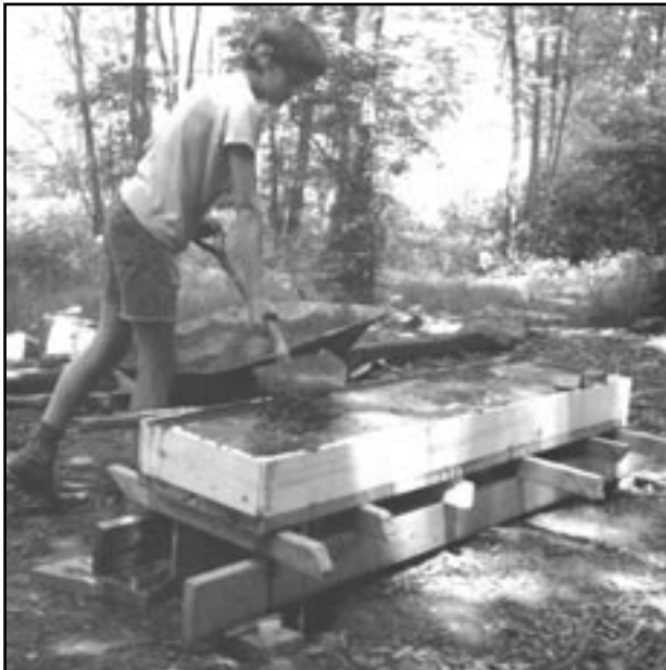
(above) Bob Schott pouring cement in 1974 for Nature Center bench.
