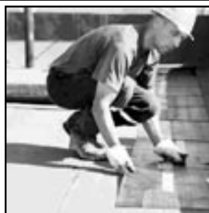
FLAT TOP ROOF
