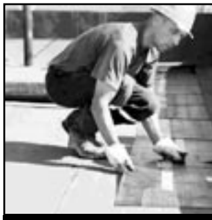
FLAT TOP ROOF
