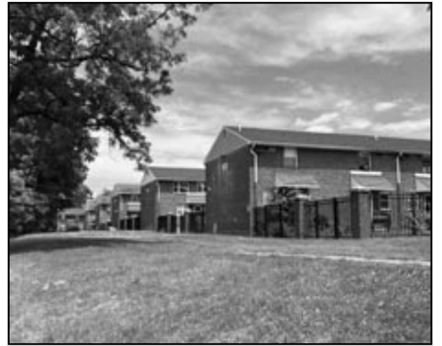
(above) Familiar sights along Leesville Avenue since 1951-52, the 17-building complex is scheduled to be razed and replaced by modern apartments.
